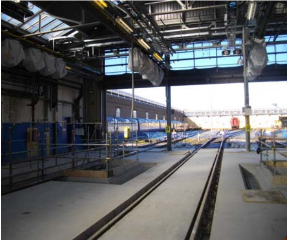
Ruislip depot shed conversion completed
