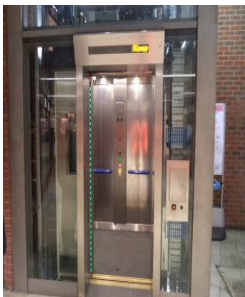
Completed lift at West Ham station
