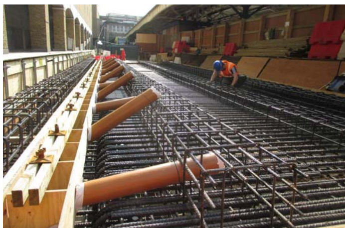
Platform track slab laying at Wimbledon station
