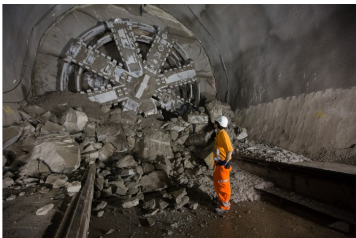
Tunnelling machine Victoria arrives at Liverpool Street – March 2015
