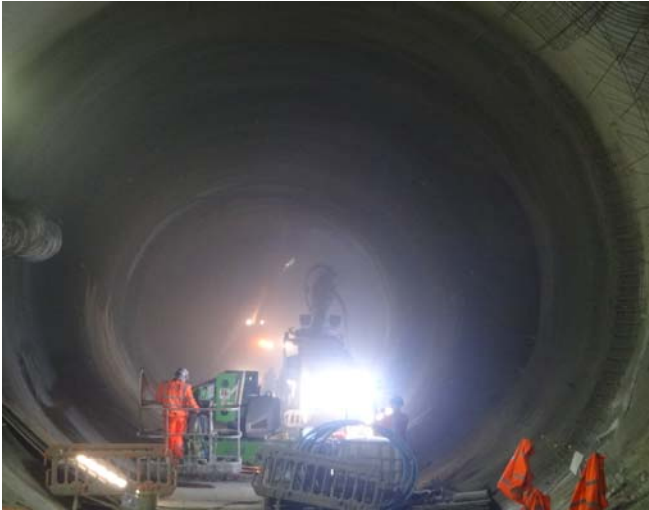
Bond Street tunnelling
