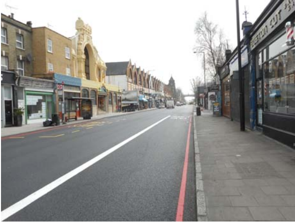
A1 Archway road carriageway resurfacing
