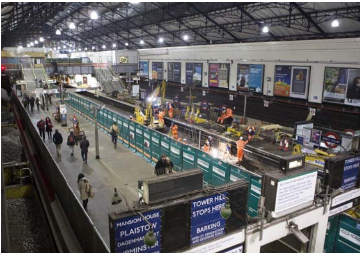
Track renewal at Earl's Court during a major closure
