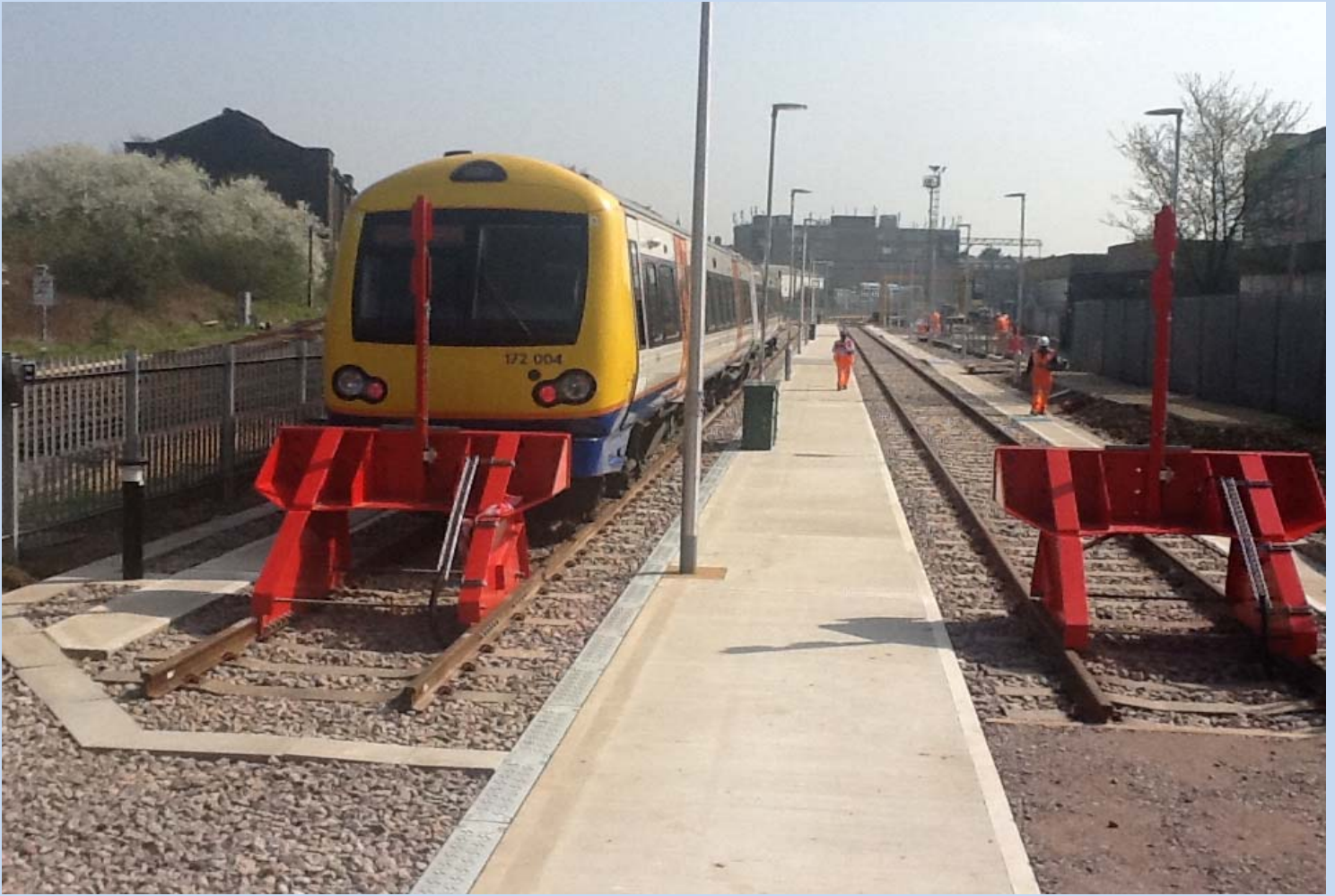
Photo: Willesden ready for five car configuration
