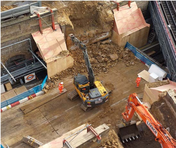
Whitechapel Station Winthrop St bridge removal
